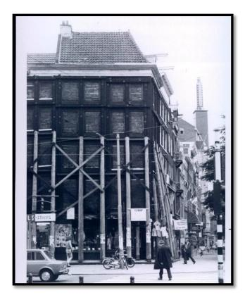
My travel photo shows a building in Amsterdam, 1973, propped up by large poles and braces, yet still functioning, with people shopping and working inside. It looks like it is still possible to save the building with proper new supports – steel I-beams and such – if the work is done swiftly and carefully.
